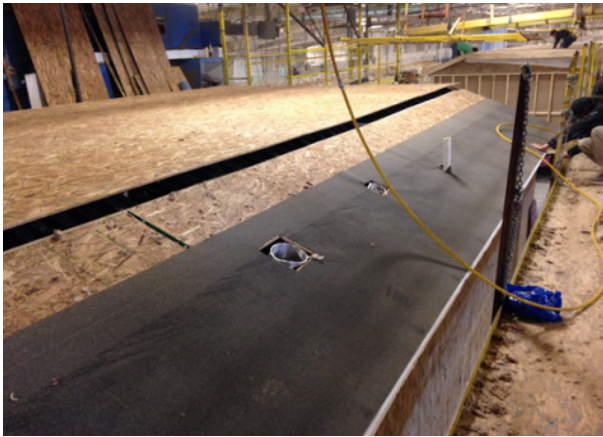
Figure C-26. Dense-packing blown insulation at eaves
