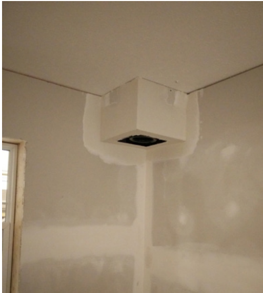
Figure C-30. Transfer fan soffit completed except for grille
