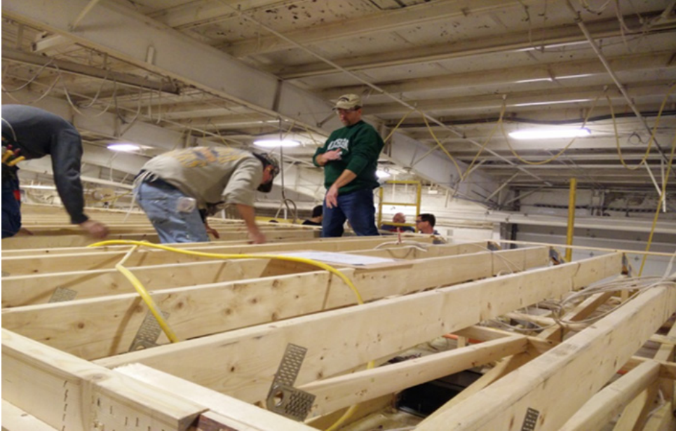
Figure C-24. Plant electrical workers route wiring above ceiling
