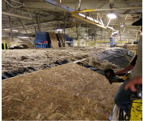
Figure C-27. Rooftop OSB decking laid over vent channel material
