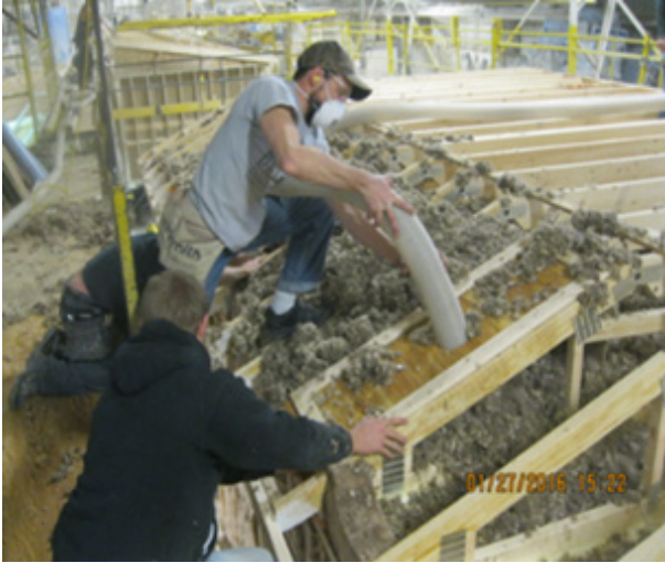
Figure C-26. Dense-packing blown insulation at eaves
