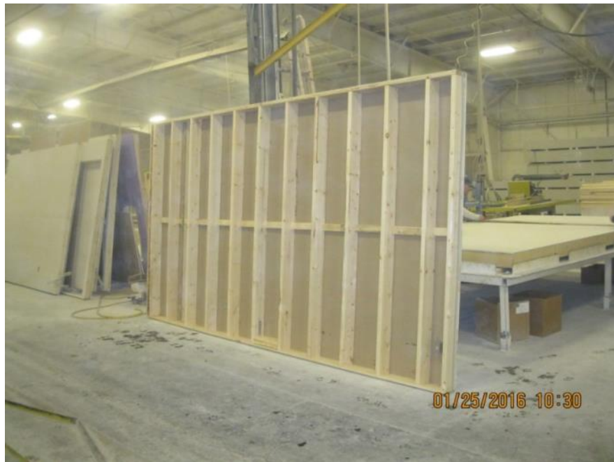
Figure C-12. Wall build station
