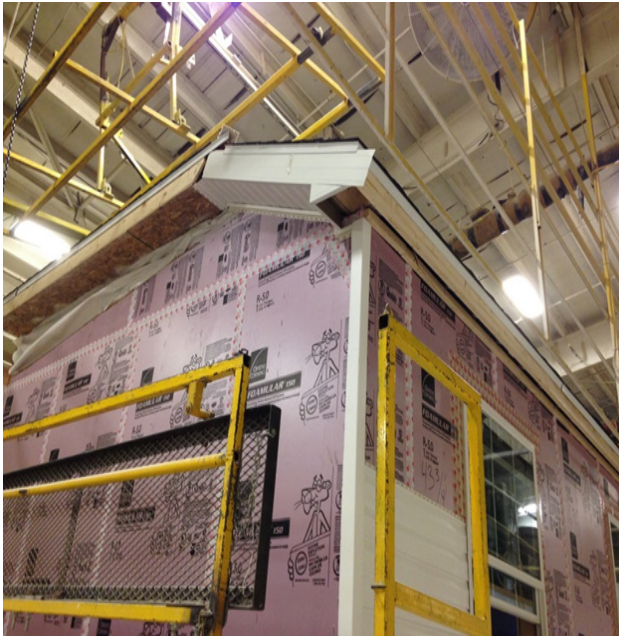
Figure C-34. Vinyl siding and soffit installation
