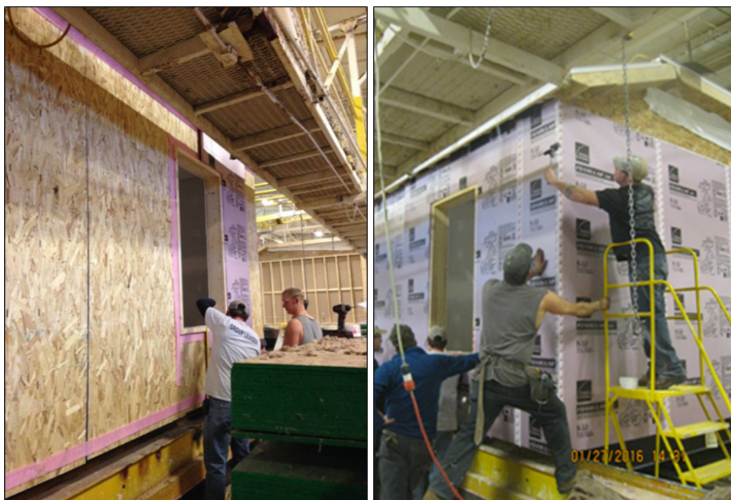
Figure C-22. Owens Corning RimSealR foam gasket is stapled to OSB wall sheathing (left); Rigid foam insulation is stapled to sheathing and taped with Owens Corning HomeSealR Tape (right)
