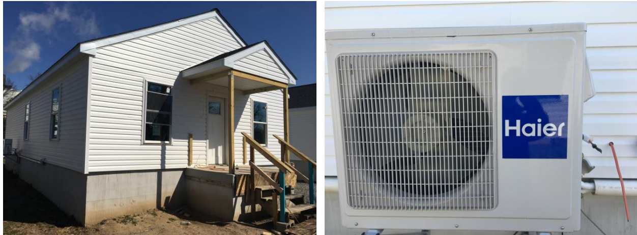
Figure 66. Maryland home street elevation (left); heat pump (right)
