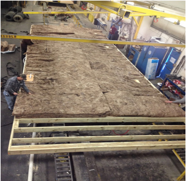
Figure C-7. Slicing blanket insulation in outrigger areas
