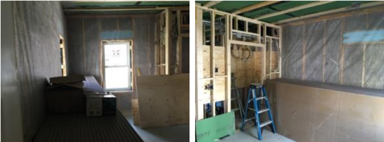
Figure 50. Blown-in cellulose insulation at Grade I level quality
