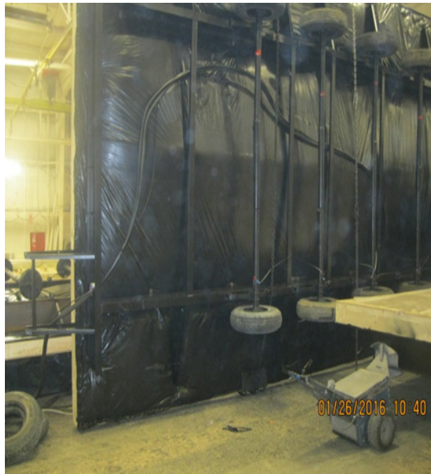
Figure C-10. Floor assembly being lifted (refrigerant lines for heat pump are visible under the floor)
