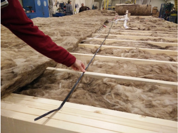
Figure C-5. Plastic strapping to hold batts in place
