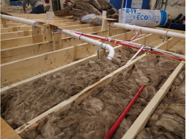
Figure C-4. Batts being laid into joist cavities
