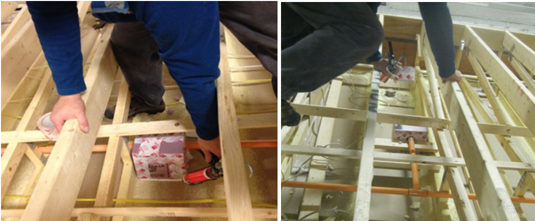
Figure C-25. Ceiling sprinkler penetrations air-sealed with rigid foam boxes and caulk
