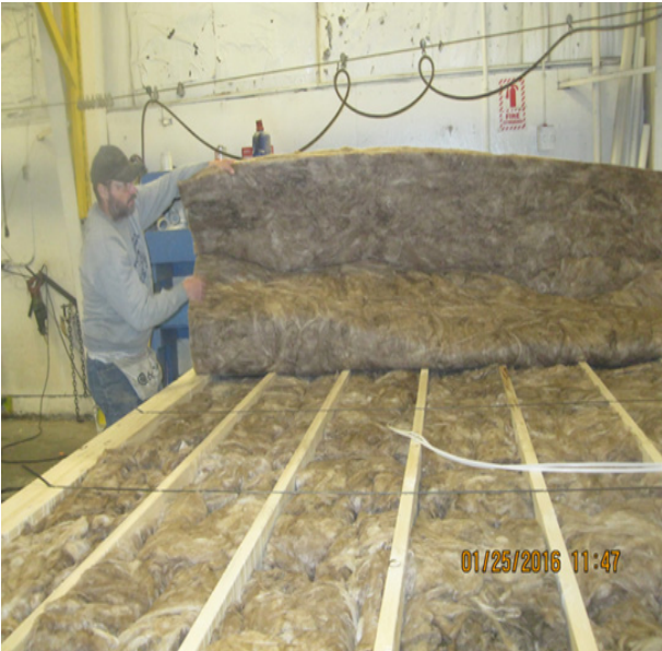
Figure C-6. Rolling out blanket insulation
