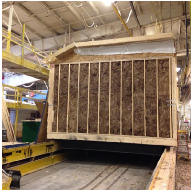
Figure C-20. View of batt insulation in exterior wall stud bays
