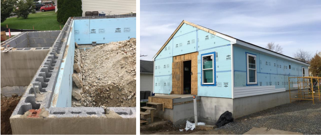
Figure 64. Maryland home foundation with vertical slab edge insulation (left); continuous exterior insulation (right)
