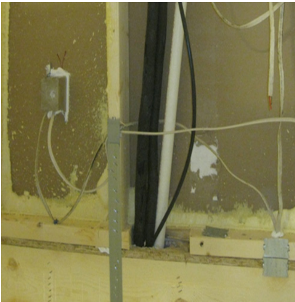
Figure C-19. Electrical boxes sealed from back with caulk
