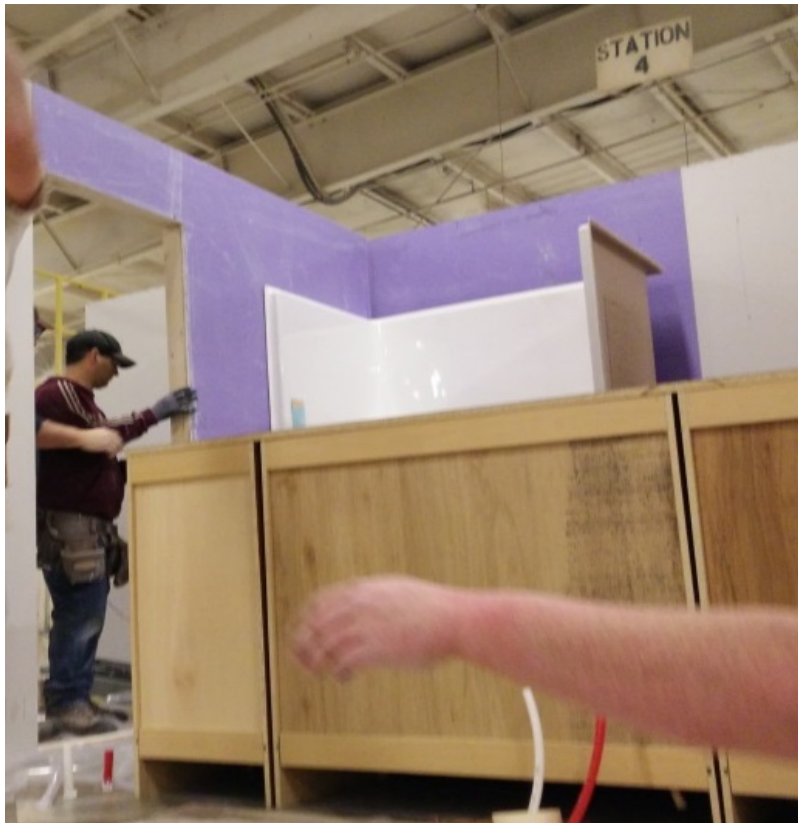
Figure C-17. Moisture resistant cement board (purple) used behind tubs
