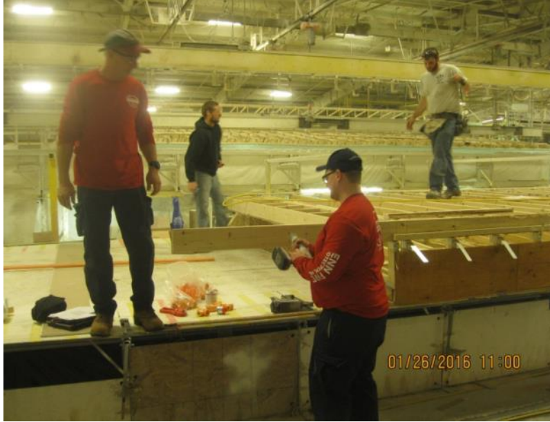
Figure C-18. Sprinkler contractors at roof table
