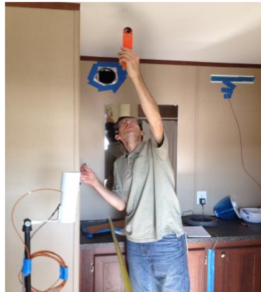
Figure 6. Measuring air speed at the master bathroom transfer fan (air outlet)
