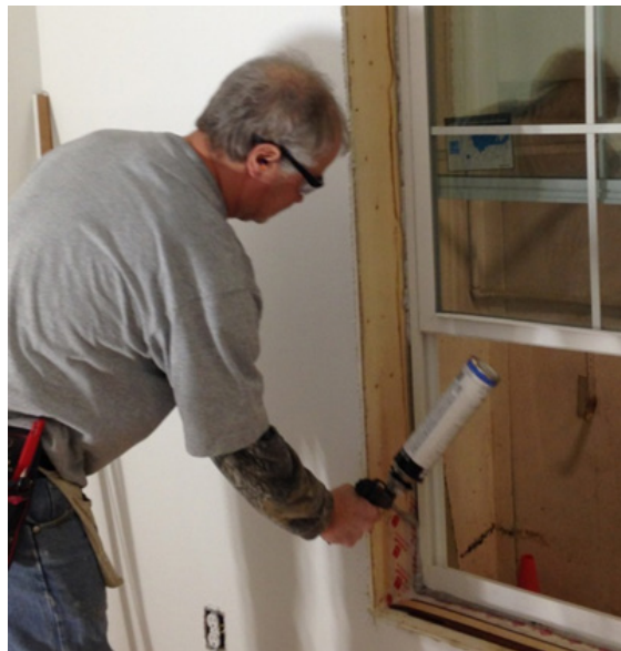
Figure C-33. Low-expansion foam being applied as interior window frame seal
